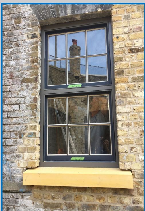
Trustees Colin & Keith installing window sills before fitting the windows
