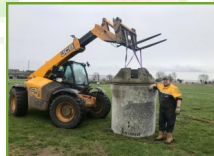
Positioning of Tett turret
