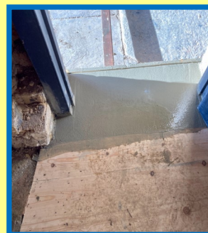
New step has been cast for the door
