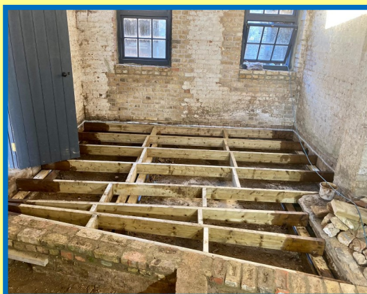
Floor starting to take shape now and a large area ready for boards
