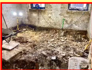
Supporting wall for joists built, base for cell walls built to floor level, both with air flow gaps. Single wall at the edges being rebuilt so floor can be laid
