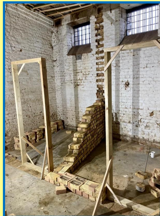
The frames for where the cell doors will be located are in situ and the brick wall between the two cells is starting to take shape.
