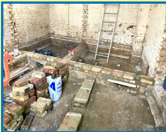
Supporting wall for joists built, base for cell walls built to floor level, both with air flow gaps. Single wall at the edges being rebuilt so floor can be laid
