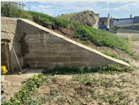
Concrete retaining wall is complete
