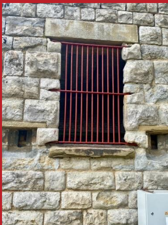
October work begins to repair broken window bars
